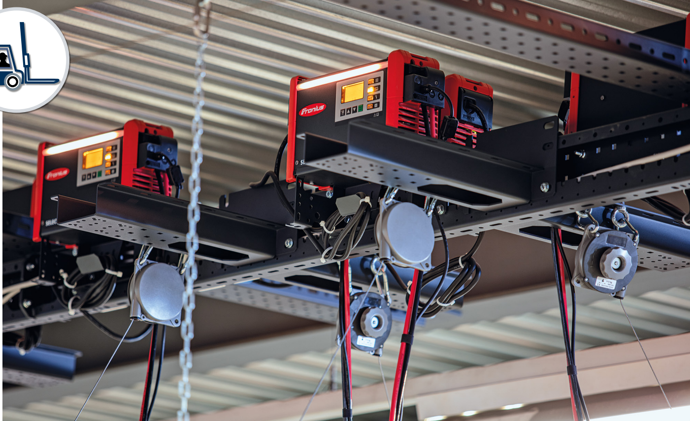
01 Fronius Selectiva battery chargers are far smaller and lighter than the 50 Hz devices previously used and allow a flexible and space-saving approach to installation
