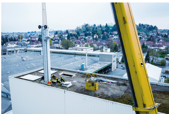
04 With energetic support from the company fire brigade, the old storage and retrieval machines were removed through hatches in the roof, and the new machines were installed
