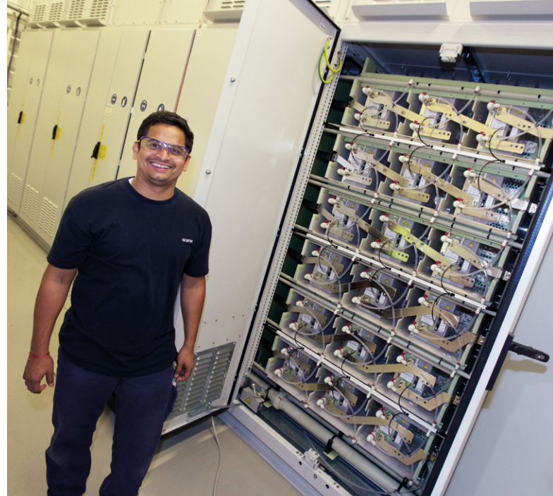
02 Sinamics SM120 CM showing the cell frame for uninterrupted operation
