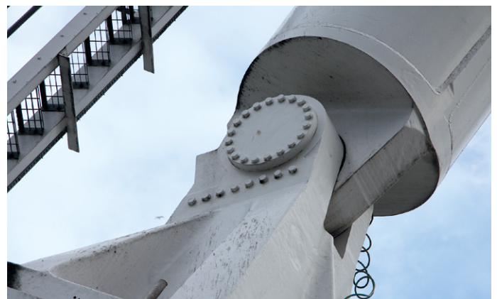
05 Two Elges bearings equalize the wind loads
