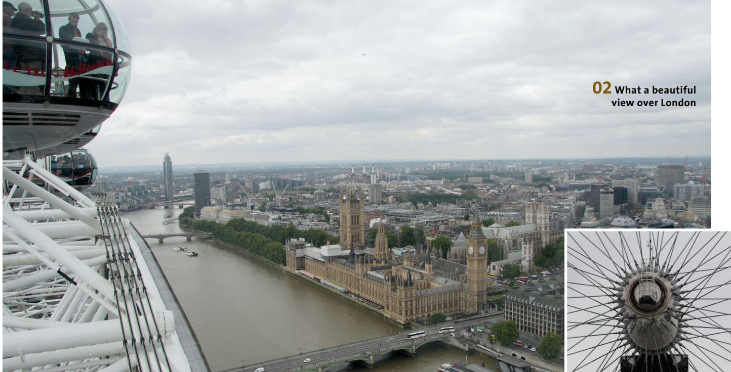
03 The hub is introduced with self-aligning roller bearing
