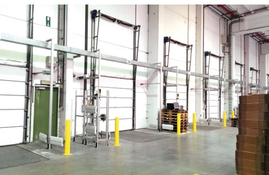
Each truck is equipped with an RFID-Gate in order to clearly document the loaded pallets
